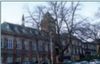
Queen Elizabeth Sixth Form College, by Hoskins, is a significant local building making a positive contribution to the Conservation Area.
