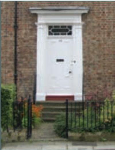
Doorway featuring pilasters and entablature with fanlight above. Note the raised ground floor and steps up to the entrance, at the end of a direct path to the street.
